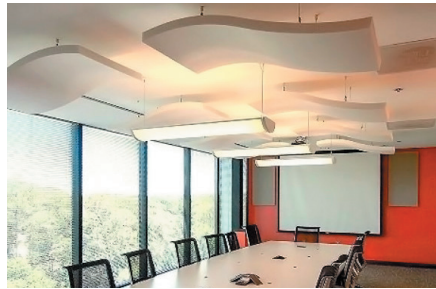
Credit: Acoustical Solutions Lighting and acoustic clouds battle for space, making for a lot of clutter in the ceiling
