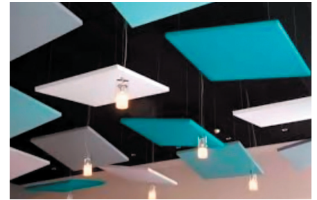
Credit: Dox Acoustics A creative approach to acoustics limits the options available to provide general illumination within a space
