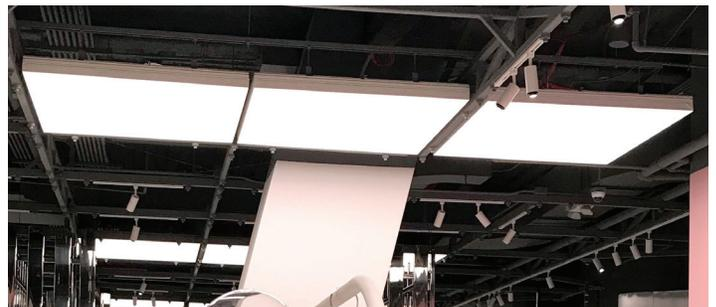
the visual clutter created when trying to combine luminaires for general lighting in the same space as the sound absorbing fixtures.
