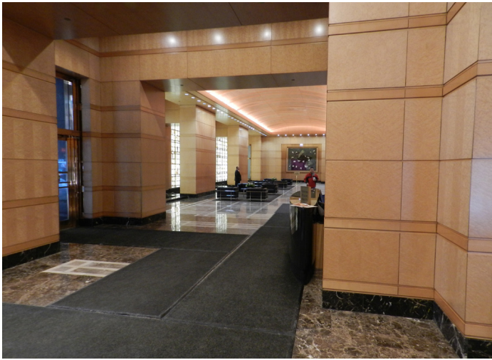
Lobby prior to renovation with subdued illumination
